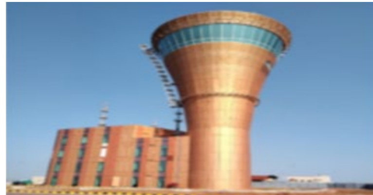
MOPA International Airport, Goa India
